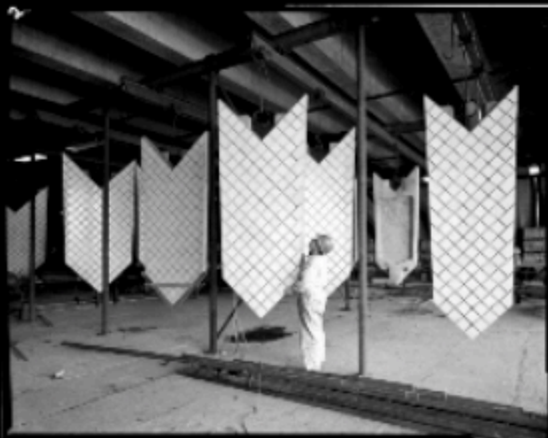
Roof tile panels
