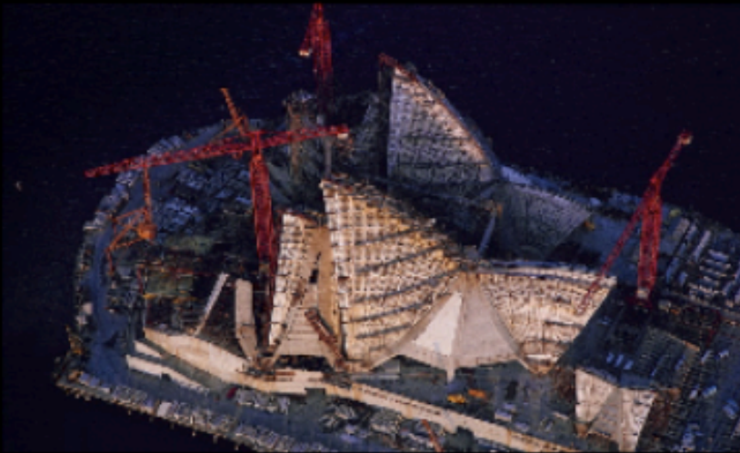
Stages 2 & 3 Roof & Interiors Hornibrooks
