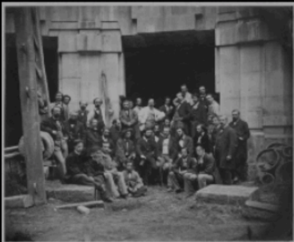
Garnier with construction crew
