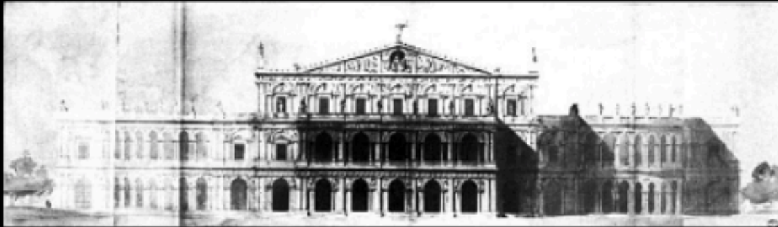
Charles Rohault-de-Fleury official Govt Architect Helped prepare the brief.
