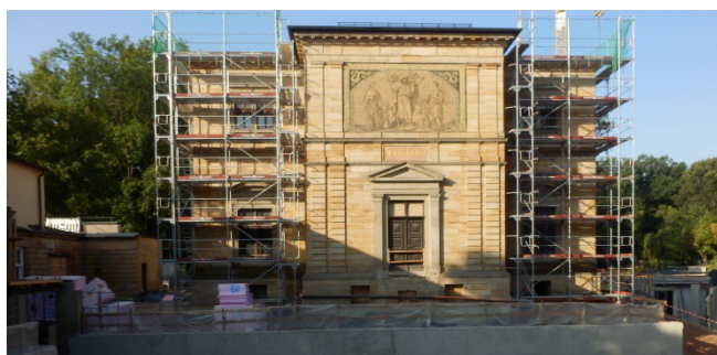
Excavation in front of Villa Wahnfried – possibly for the Archives
